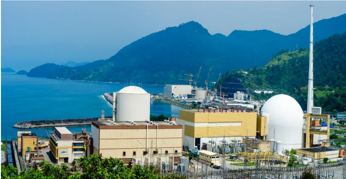
Figure 2: Site view of Angra NPPs
