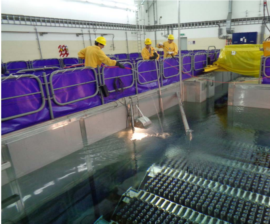
Figure 6: Ultrasonic system installation with operator assistance in CNA1
