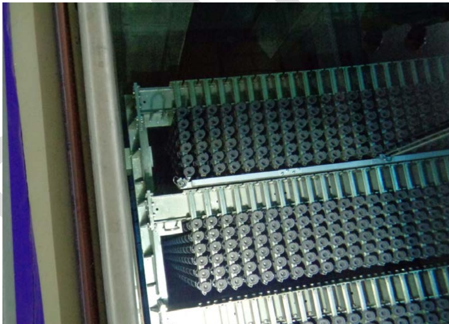
Figure 7: Close view of sealing bar of hangers into the pond
