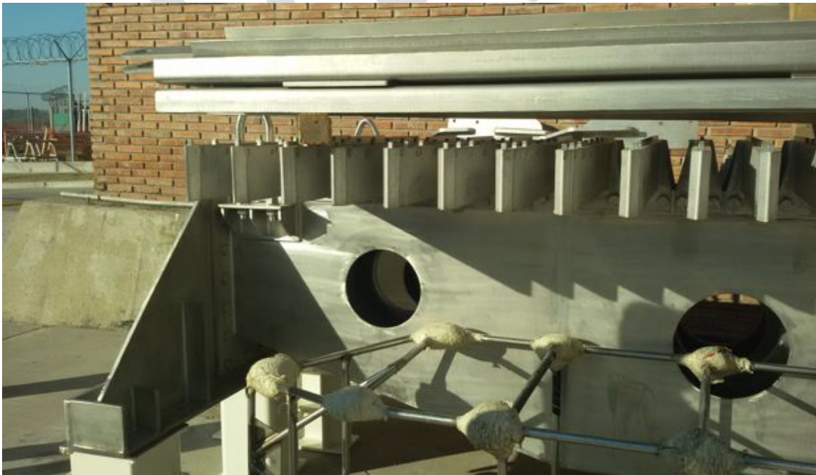
Figure 4: View of the hangers outside of the pond
