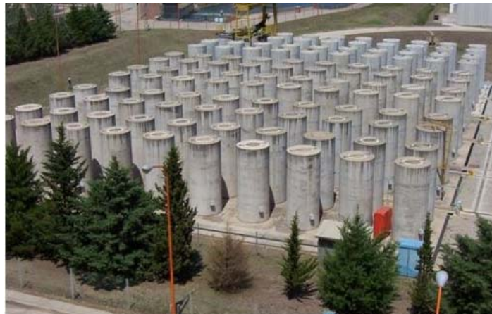
Figure 1: The modular array of concrete silos (dry storage) at Embalse.
